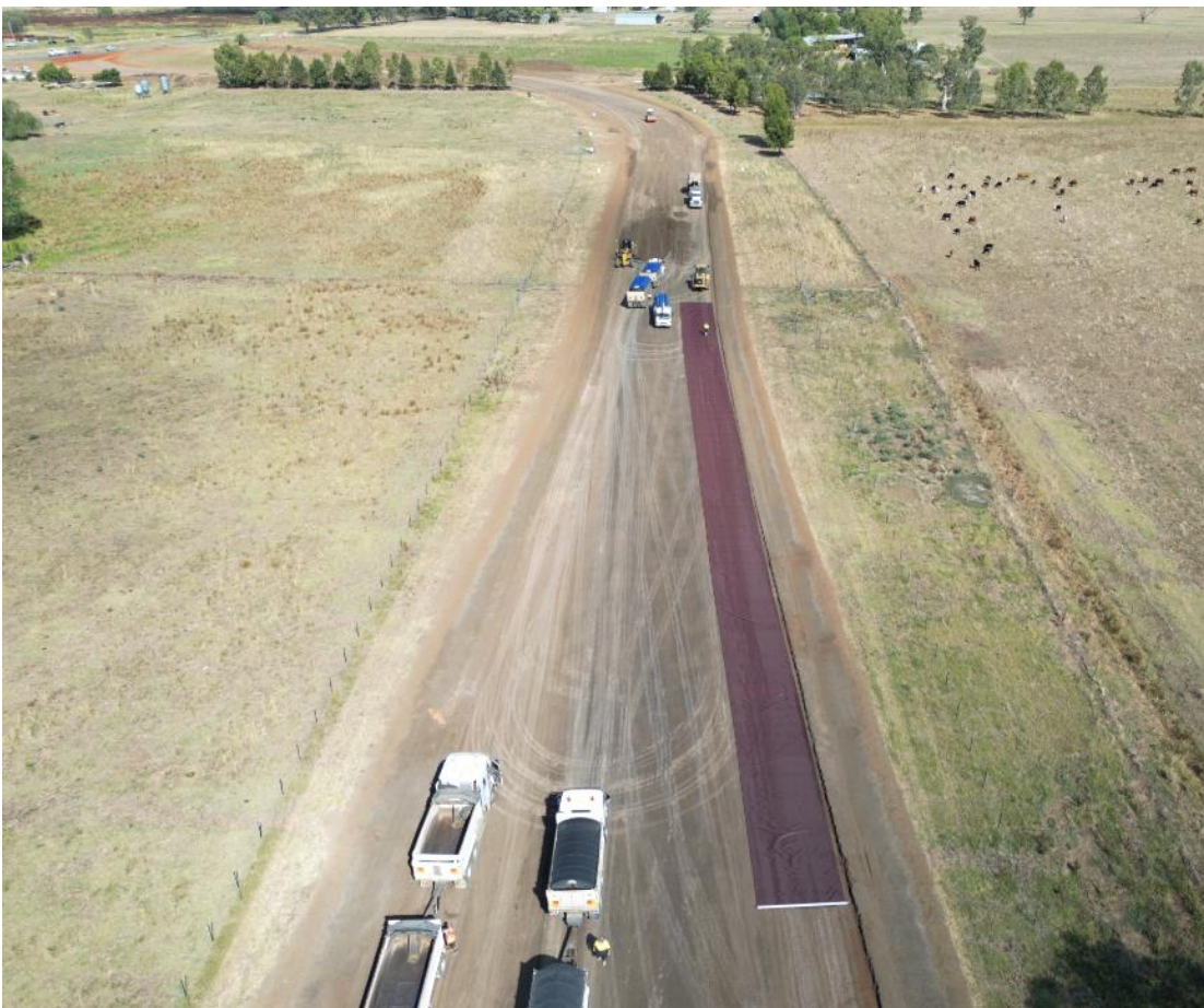
Figure 4 – One treatment option involving the installation of high strength geotextile fabrics utilised in areas of the flood plain to facilitate pavement construction over unsuitable subgrade.
