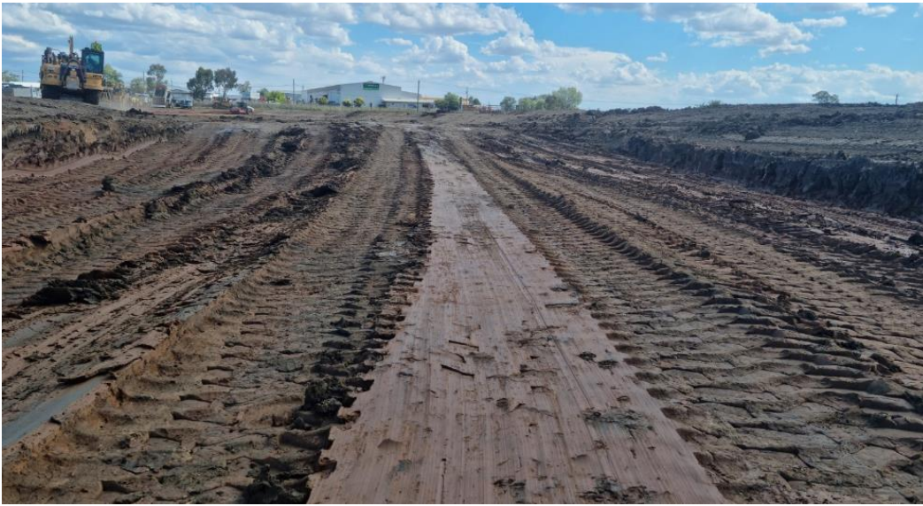
Figure 3 – Typical unsuitable subgrade within the flood plain requiring additional treatment.
