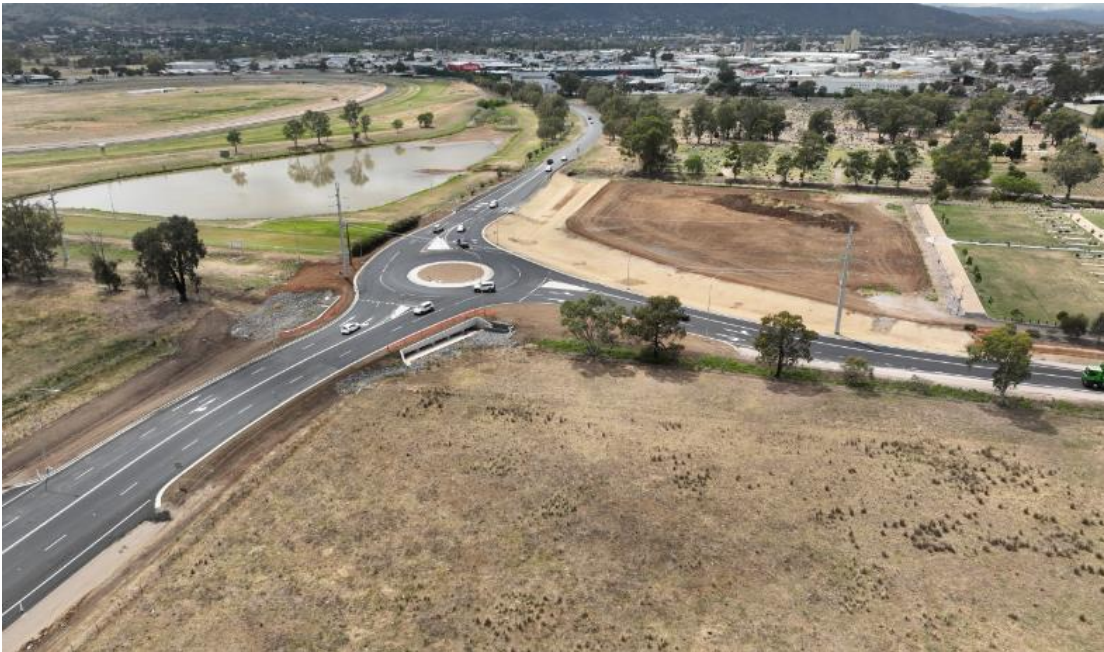
Figure 1 – Roundabout constructed at the corner of Jewry Street and Dampier Street, with the Jewry Street extension bypass on the left-hand side extending across the flood plain to the west (view is to the northeast).
